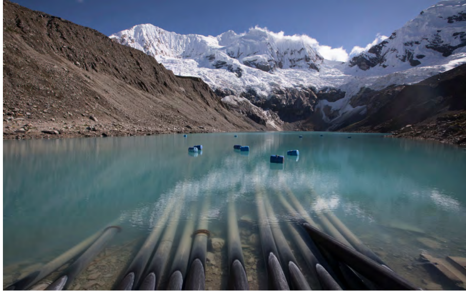
Glacial Lake Palcacocha poses significant flood hazard downstream to communities in Huaraz. Siphons installed in 2011 lowered the level of the lake by 7 to 16 feet in an attempt to reduce the flood hazard. Felipe Fittipaldi for The New York Times
